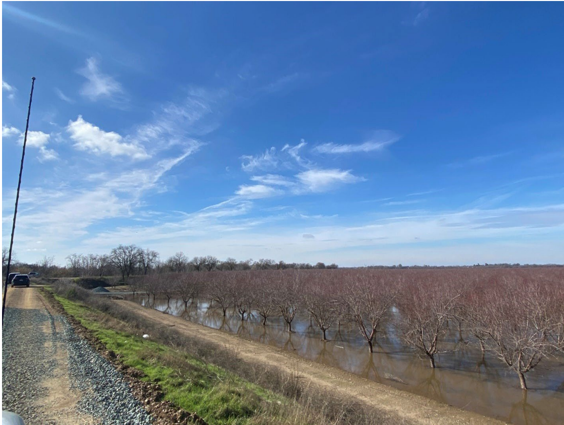
Figure 3 - As we pursue relief, recovery, and future sustainable adaptation, it will take a Herculean effort and close coordination between many jurisdictions and authorities to prevent more flooding in the future.
